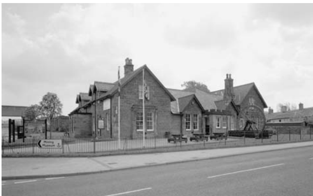
Figure 4.26: Lady Victoria Colliery, 1998. The former offices of the Lothian Coal Co. Separated from the pithead by the A7 trunk road (from Edinburgh to Carlisle), and used latterly as the offices of the Scottish Mining Museum. The building also houses the museum's excellent library and archive. SC894269
