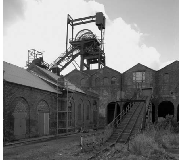
Figure 4.6: Lady Victoria Colliery, 1988. View from north west showing headgear, part of the north side of the pithead complex, and to the left, the old engine house originally used to house the temporary winding engine during the sinking of the shaft in the early 1890s. SC758215
