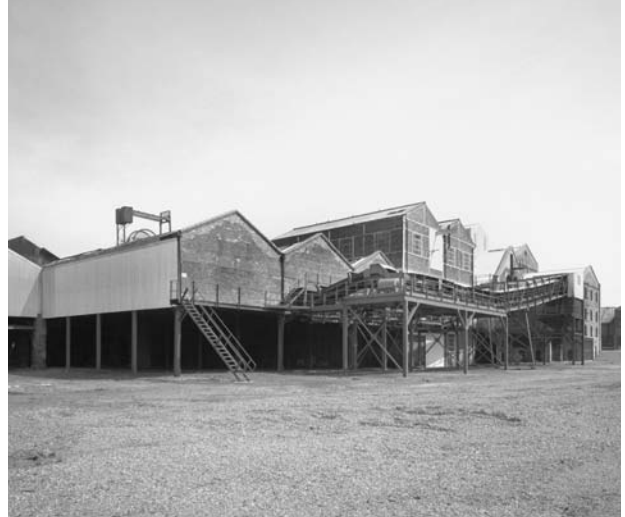
Figure 4.16: Lady Victoria Colliery, 1998. View of the south end of the colliery, showing the Dense Medium Plant (centre), which was constructed in 1963-4. SC894661
