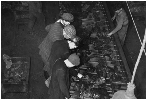
Figure 4.15: Lady Victoria Colliery, 1951. View looking down onto one of the picking tables. Sodium lighting was installed by the General Electric Company Limited in the 1950s because it made the coal glisten, in sharp contrast to the dull surface of the waste and dirt. SMM:1996.0861, SC384753
