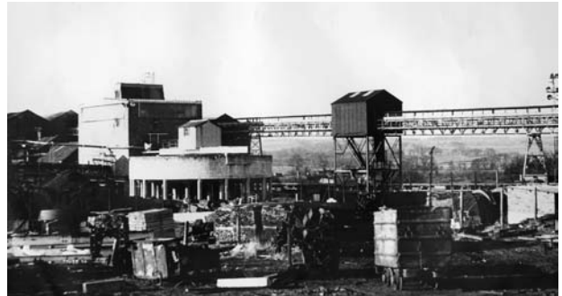
Figure 4.32: Lady Victoria Colliery, c.1965. View of the Fines Treatment Plant and Thickener, the construction of which in 1963-4 coincided with the installation of the Dense Medium Plant at the south end of the colliery. SMM:1996.0666, SC384760
