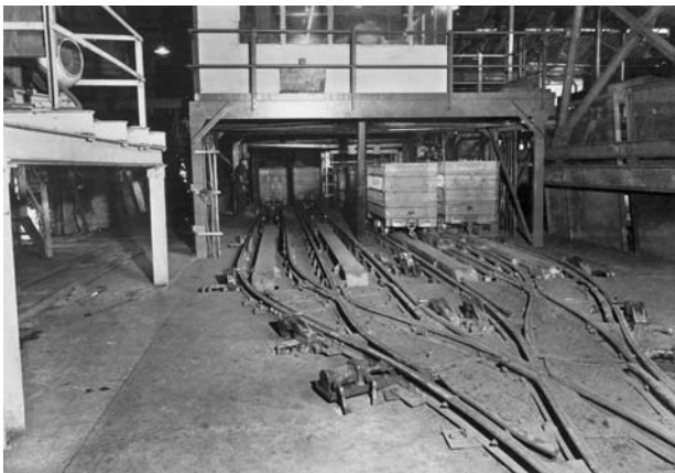
Figure 4.14: Lady Victoria Colliery, c.1981. View of the tub circuit and banksman's cabin, situated close to the top of the shaft, from where operations at the pithead were controlled. SMM:1997.0548, SC382549
