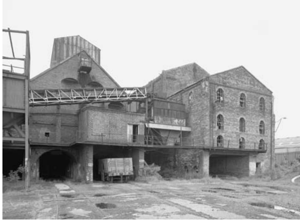
Figure 4.18: Lady Victoria Colliery, 1993. View of the south-east end of the colliery showing the cross Hopper (left) and the Old Washer (right). SC894265
