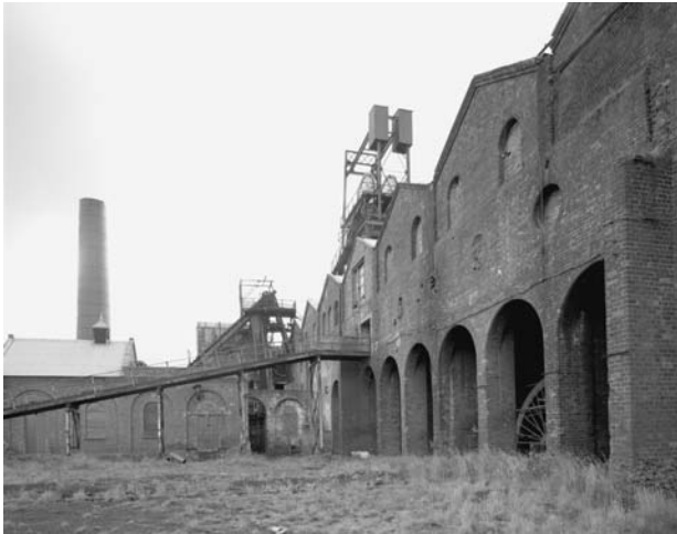
Figure 4.30: Lady Victoria Colliery, 1988. View of the 'Dredger', situated between the boilerhouse chimney (left) and the headgear (right). Its function was to extract by means of a bucket elevator coal dross at the bottom of a settling tank containing water from the old Washer, the dross being used to fuel the boilers in the adjacent Boiler house. SC894668
