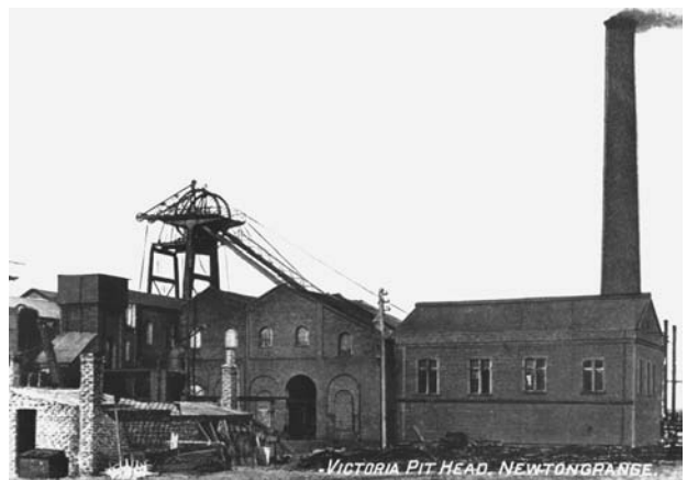
Figure 4.33: Lady Victoria Colliery, c.1895. This view shows the pithead shortly after the colliery came into production, and before the addition of other buildings around the pithead, including the Old Power Station. SMM:1997.0980, SC382551
