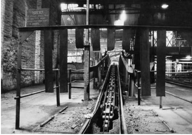
Figure 4.13: Lady Victoria Colliery. View of the 'creeper', which, after gravity had taken the tubs (or hutches) to bottom of the tub circuit, brought them back up to its summit at the pithead. SMM:1997.0893, SC382550
