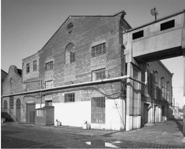
Figure 4.24: Lady Victoria Colliery, 1991. The New Power Station, before its conversion to house new museum exhibition areas and visitor facilities. The gantry to the baths can also be seen (top right). SC894669
