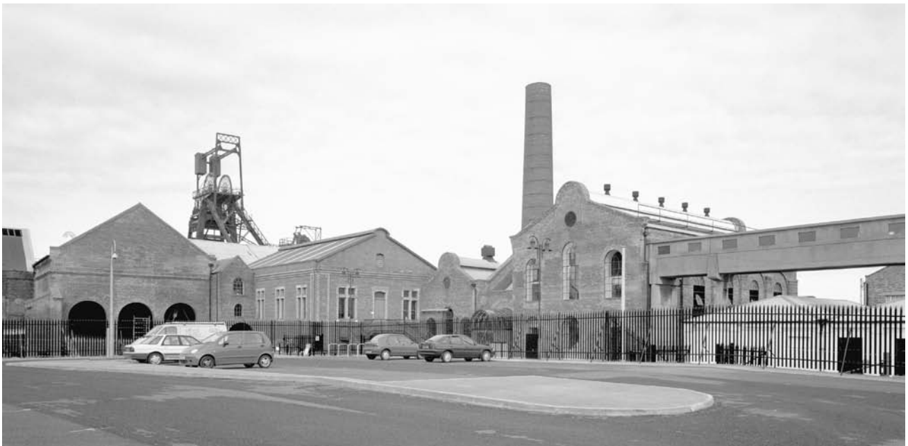
Figure 4.31: Lady Victoria Colliery, 1999. View of the pithead in 1999 after the completion of a £5 million renovation and redevelopment programme by the Scottish Mining Museum. SC894268
